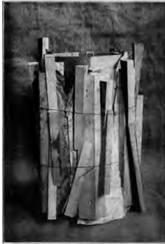
Fig. 256. Gluing up a Column Joint. (Pinch-Dogs at Top of Joints.)
