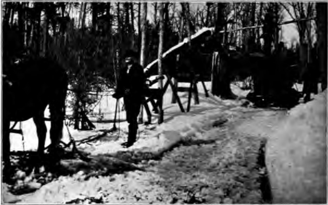
Fig. 10. Making an Ice Road by Flooding.
