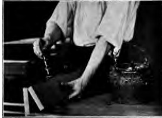
Fig. 260. Applying Glue for an Edge-to-Edge Joint.
