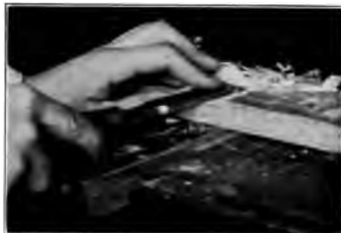
Fig. 71. Chiseling Out a Dado (Second Step).
