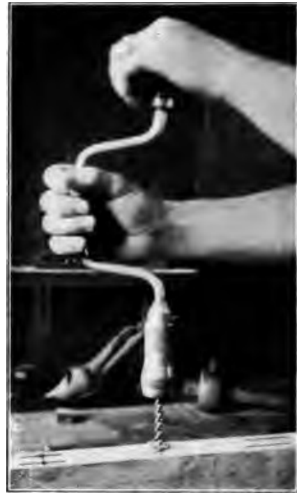
Fig. 263. Boring for Dowels in an Edge-to-Edge Joint.
