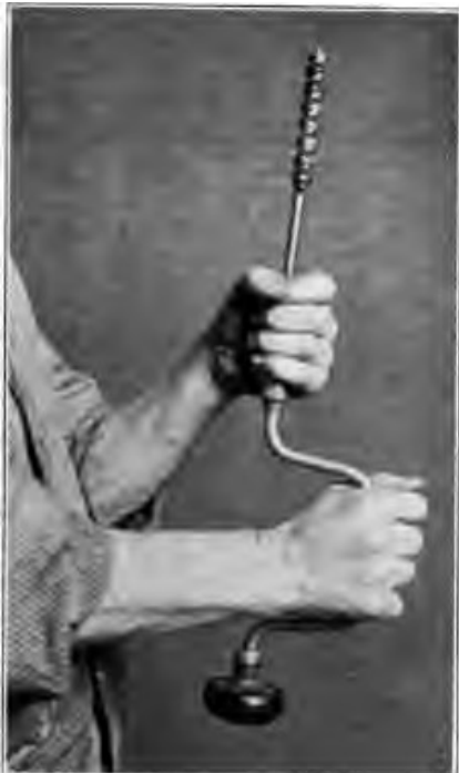
Fig. 186. Inserting a Bit in Stock.
