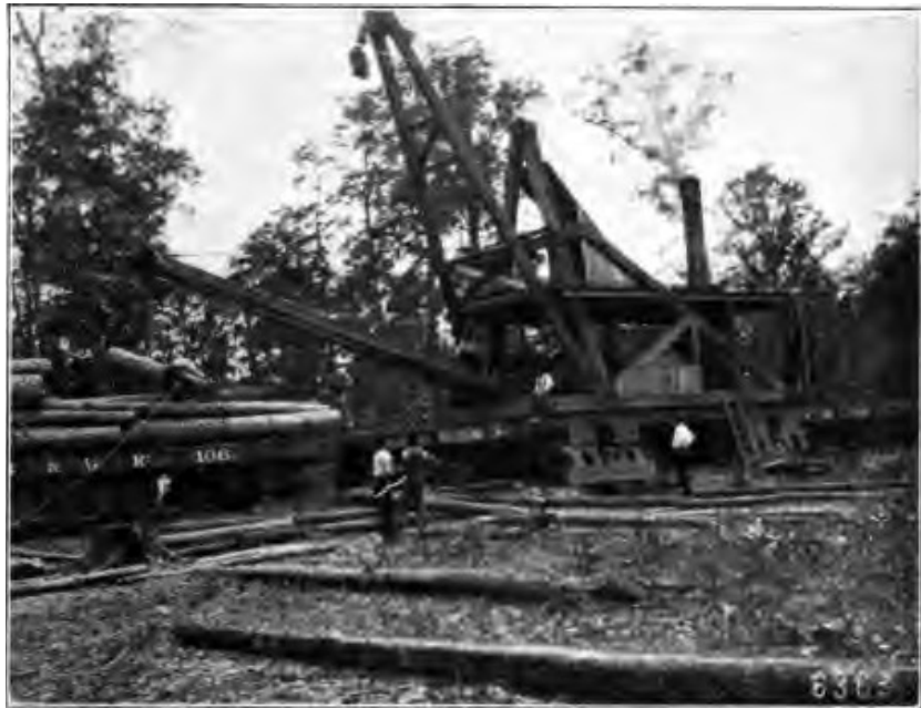
Fig. 27. Steam Skidder at Work. Grant County, Arkansas.
