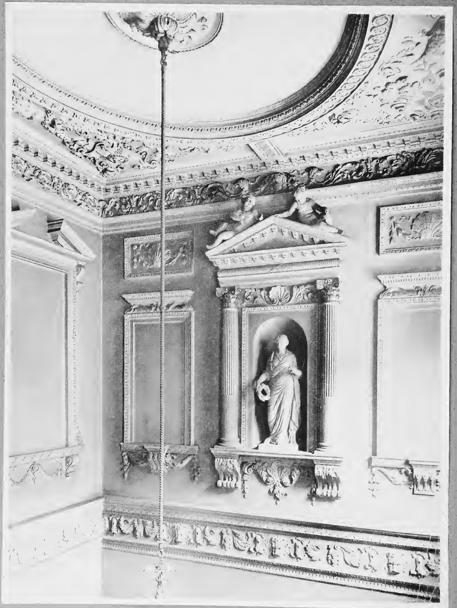
PLASTER DECORATION, UPPER PART OF HALL AT 30 OLD BURLINGTON STREET DESIGNED BY WILLIAM KENT
