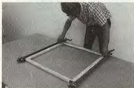
Measuring length of mullion
