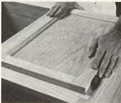
Positioning door over opening
