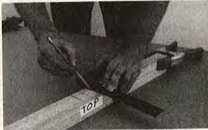
Marking position of mullion
