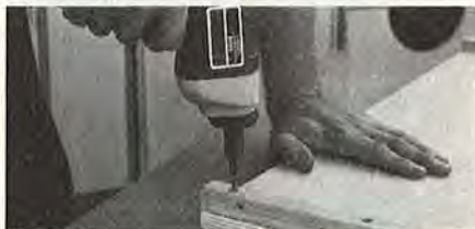
Fastening cleats to end panels
