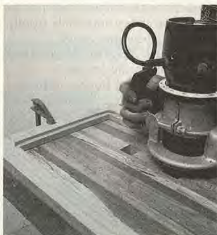
Routing back side of door
