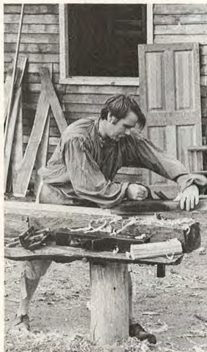
The adjustable plow plane is an essential tool of the joiner.
