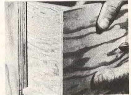
One of the simplest methods of drawer-and-guide construction which can be made with power tools. The drawer slides in slots dadoed into the 3/4" plywood cabinet sides. (American Plywood Assn.)
