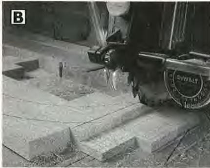
B Dadoing the arch top half-lap joints
