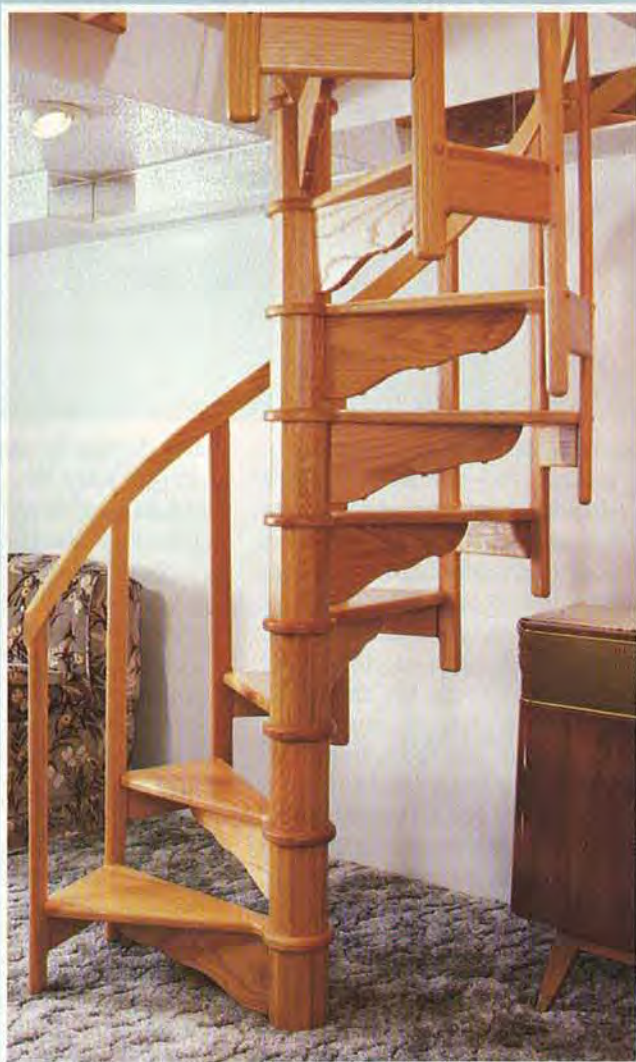
In his home, Carmen exhibits the craftsmanship he teaches. He built this solid red oak spiral staircase between the living and recreation rooms. The rail, made of 1/4" laminated strips, was bent in place on the staircase.
