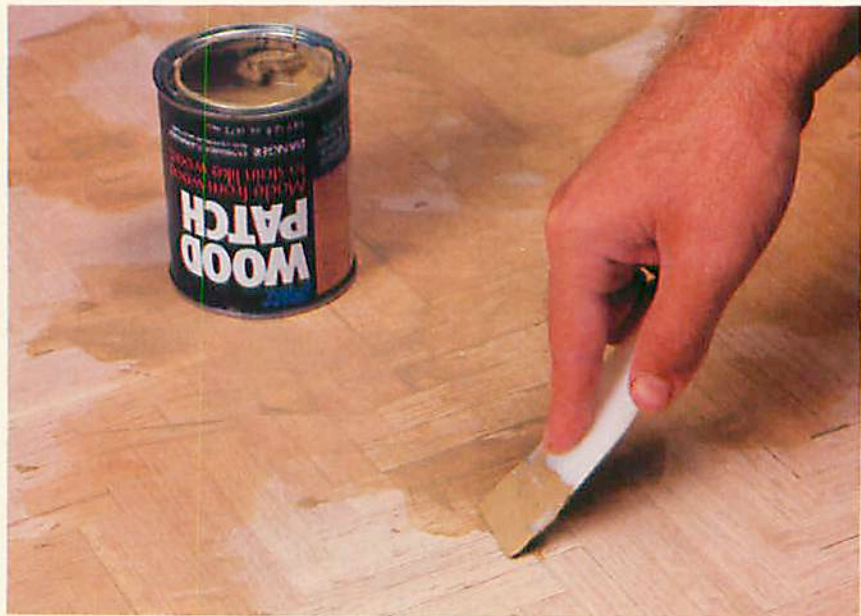
We used FIX oak-colored wood patch to fill the cracks between the oak strips on our tabletop. Force the wood filler into the cracks with a putty knife.
