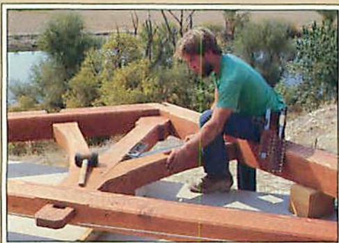
Sam assembles a king-post strut on the end section of the timber frame.
