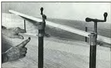
Using a penny as a spacer for an even overhang, glue and clamp the stiles to the cabinet front.
