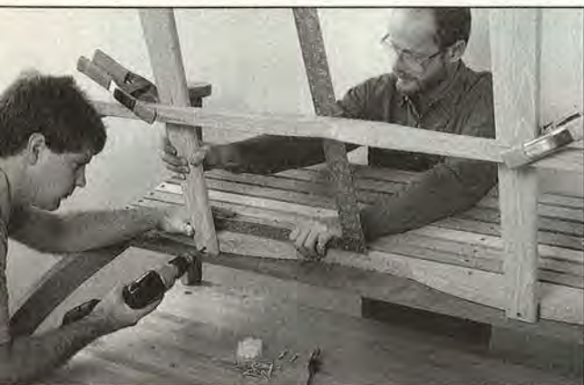
Align the top and bottom supports, position the center slats, and fasten them to the supports.
