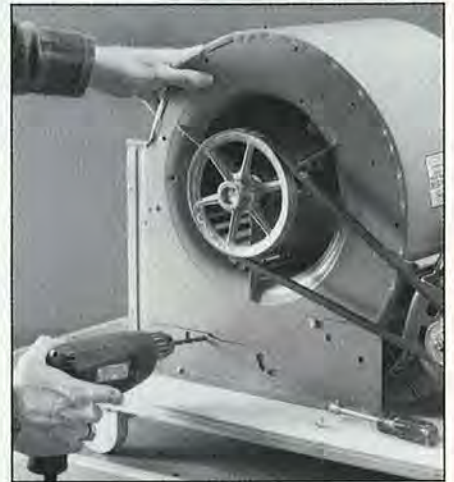
Drill holes into the blower housing, using the existing holes in the blower bracket as guides.
