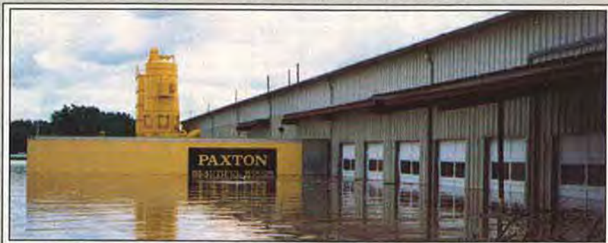
In July 1993, surging water from the Raccoon River in Des Moines, Iowa, flooded the Frank Paxton Lumber Co. yard (loading dock shown) and other businesses.
