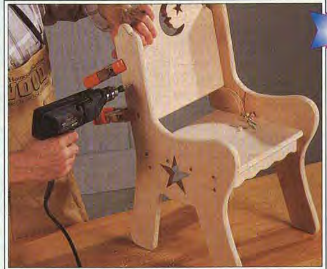
Glue and screw the backrest, stretchers, and seat between the chair sides.
