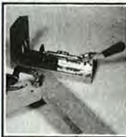
3) Drive self-tapping screws.
