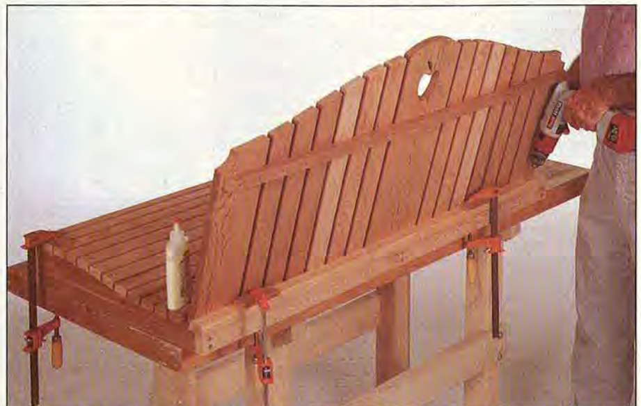
Clamp the backrest assembly to the seat frame, drill countersunk mounting holes, and screw the backrest bottom cleat to the seat-frame rear crossmember.
