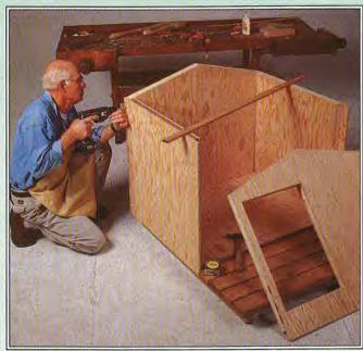
Screw the side panels to the floor and back panels. A scrap strip helps hold the side panels upright and square.
