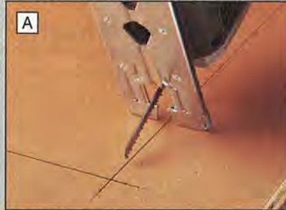
To start the plunge cut for the window, position the jigsaw on the plywood with the blade not touching the wood but centered over the cutline.
