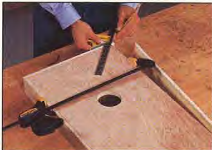
Use a combination square to mark the miter cutlines on the pieces that surround the top plywood panel.
