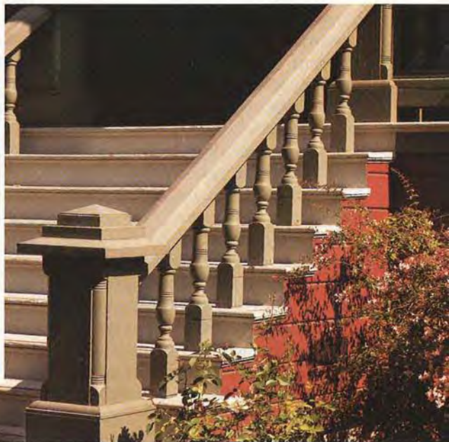
Below: Gail turned hundreds of Victorian balusters for Oakland's Preservation Park. The entry stairs of the Remillard House display another one of the many styles of turnings used in the Victorian era.
