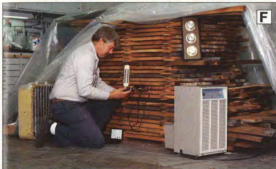
F During the dehumidification-drying process, I check relative air humidity and temperature daily. I periodically uncover the stack to check the wood moisture content.
