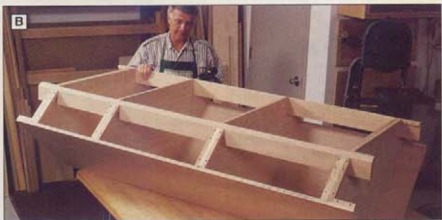
B Secure the notched supports to the previously installed shelves by driving wood screws through the previously drilled cleats.
