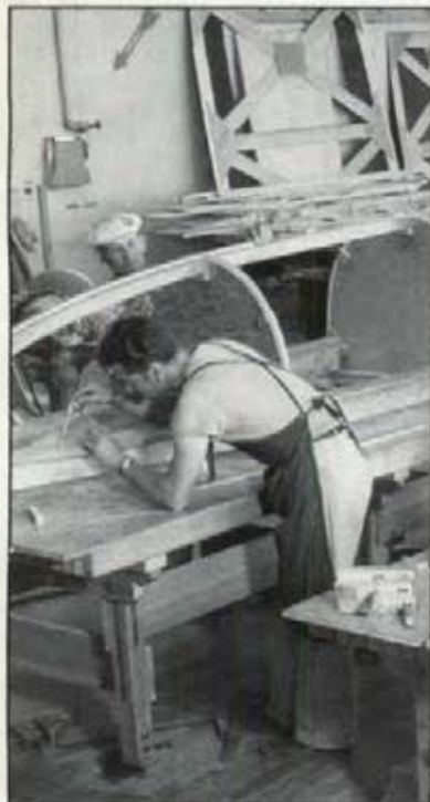
Workers in Howard Hughes' Culver City, California, hangar build what appears to be pontoon pods for the HK-1 flying boat.
