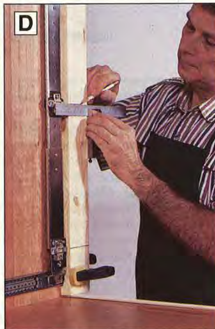
D Transfer the hinge hole centerpoints to scrap stile, and drill the holes to verify hole locations before drilling the holes in the door stiles.
