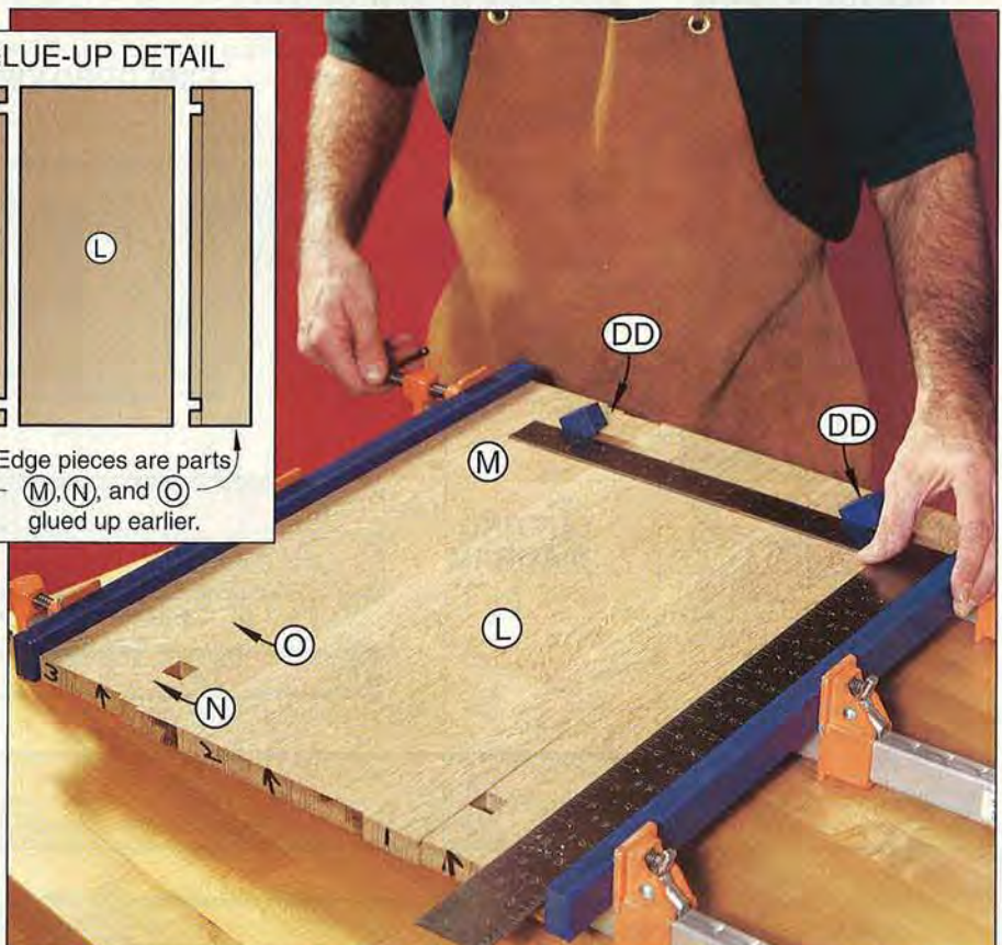
A carpenter's framing square and spacers DD help align the top's mortises to fit over the tenons on the side panels.
