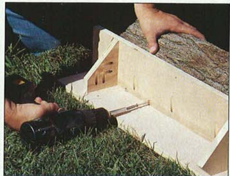
Drive a couple of long drywall screws into the log through the jig's back. The jig will act as a surrogate straightedge until you can cut one.
