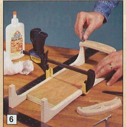
6 Clamp the bases to hold them square while assembling the carrier.
