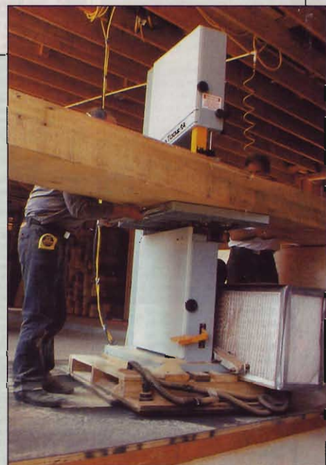
Floating on a cushion of air, the bandsaw easily maneuvers through a huge timber that will become a corbel in a custom California home.
