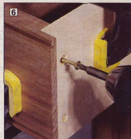
Use screws to secure the rabbet joints where the drawer rails and front rails meet.
