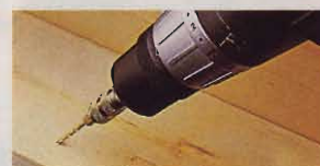
Drill pilot holes
