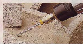
Drill into masonry
