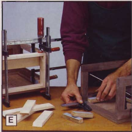
Use a combination square to accurately position the blocks. A spacer clamped across the case keeps it from spreading when the reveal fronts are glued in place.
