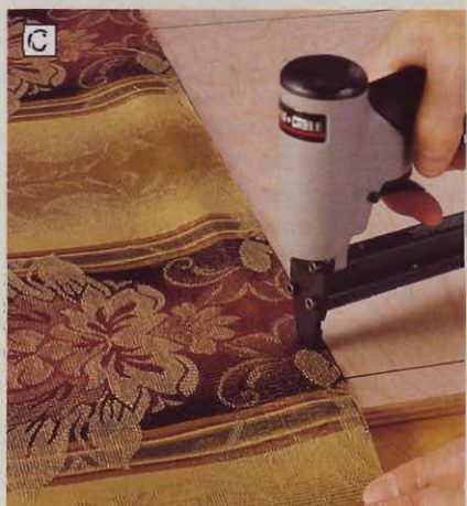
C Stop your staples 2" from the end of the ½" plywood cushion panel when tacking the fabric in place.
