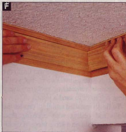
Photo F Move the other piece of molding as needed to get a perfect match with the coped piece. Pin them close to the joint.
