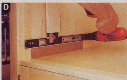
A scrapwood spacer keeps the bottom door slide perfectly aligned.
