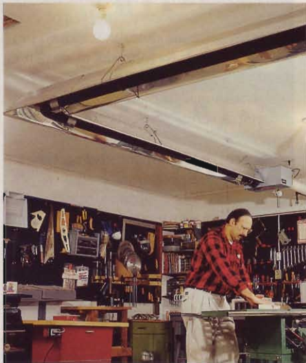
Radiant tube heaters, such as this Re-Verber-Ray unit, are available in several sizes, and can be configured in straight, "U" and "L" shapes to fit the space
