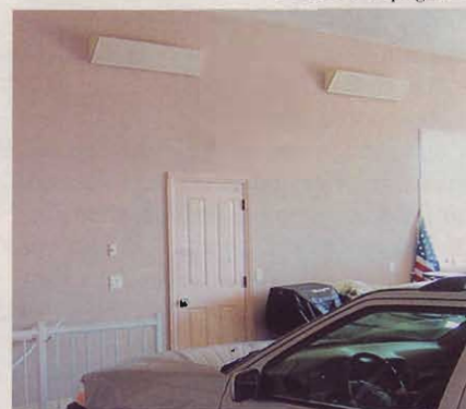
Cove heaters from Radiant Electric Heat, Inc. provide economical radiant heat without taking up much space. Heating large areas requires multiple units.
