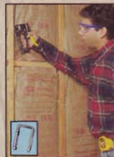
Install Insulation
