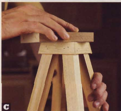
C Using a sanding block with 80-grit sandpaper, flatten the top edges of the rails (C) to receive the top assembly.
