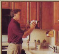
Cabinet Refurbishing - cleaning, degreasing, repairing and polishing
