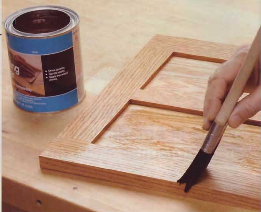
Apply sanding sealer on raw wood or over stain. Let the sealer dry, sand off the rough wood fibers with minimal effort, and add a smooth, clear topcoat.
