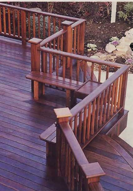
Oil finishes give ipé a deep, reddish-brown tone, inhibit fading, and hide the yellow pores.
