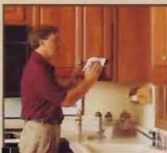
Cabinet Refurbishing - cleaning, degreasing, repairing and polishing
