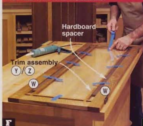
With the trim assembly (Y/Z) and spacers held tight against the glass and bottom door stiles (W), apply tape to hold the assembly in place while the caulk cures.
