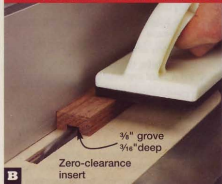
Install a zero-clearance insert in your tablesaw, and cut a 3/8" groove 3/16" deep centered in one face of the beam (B).
