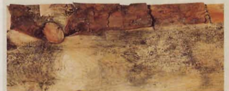
Mold, such as this, can be washed off with a water/bleach solution.
