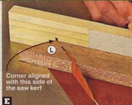
E Flip the blank, align the end of the first cut with the saw kerf, and cut a corner block (L). Flip and cut three more times.
