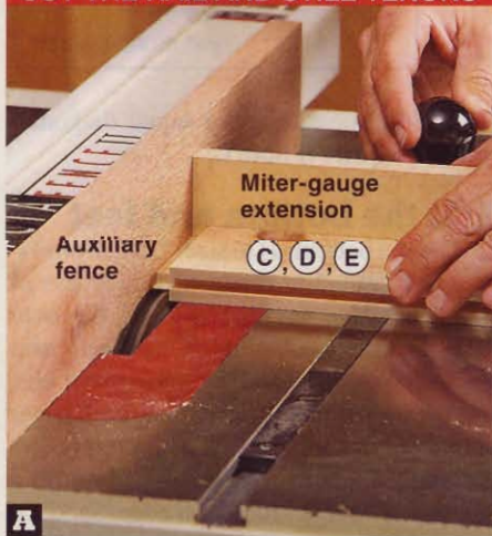
A Using a miter-gauge extension for backup, form a \frac{1}{4} " tenon \frac{3}{8} " long on each end of the rails (C, D) and center stiles (E).
