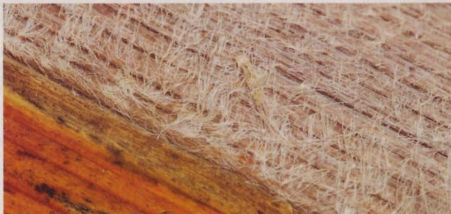
Pressure-washing this deck railing raised wispy wood fibers, a process called "fuzzing."
