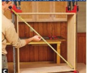
C Measuring for equal diagonals to check for square works as well for this upper case as for the lower one and the drawer boxes.
