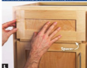
L A spacer on the door precisely positions the drawer front as you press it against the drawer box.
