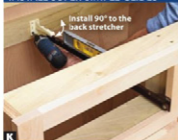
K The plastic mounting bracket lets you adjust these slides up and down and side-to-side for smooth-opening drawers.
