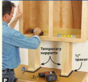
P Supports hold upper cabinets 18" above the countertop while you drive mounting screws. Spacers make the supports easy to remove.
