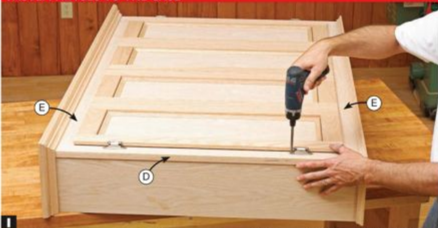
1 With rabbets on the centered double doors resting on the frame stile (D) and rails (E), drill and drive hinge screws.
