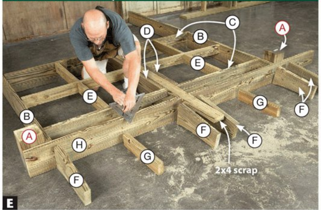
E A 2x4 in the notches aligns the crossbeams (C) and outside beam (H). Mark the locations of parts B-E on the four outside beams.
