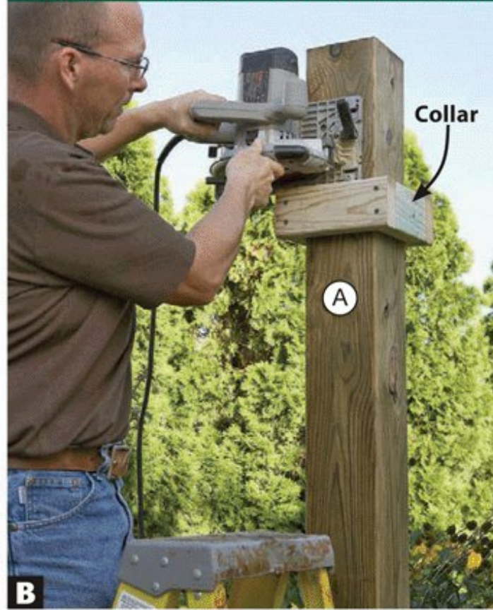
B Screw a collar to the post (A) to guide your circular saw around all four sides of the post. Complete the cut with a handsaw.
