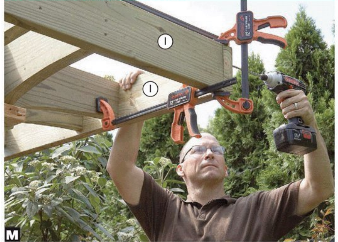
M Bringing the bands (I) together at the corners may require using clamps and spreaders to align the pieces.
