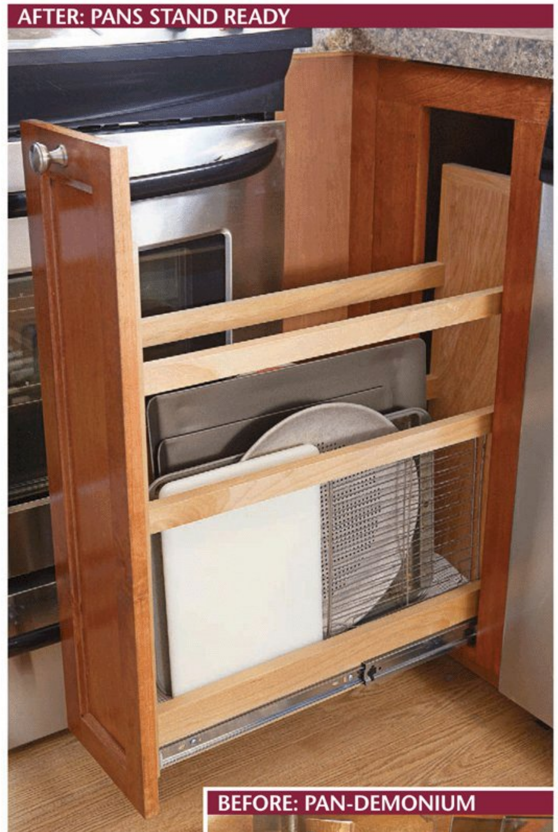
AFTER: PANS STAND READY Position the rails to support your flat pans, cookie sheets, and cutting boards. The bottom rails act as the sides of a long tray.
