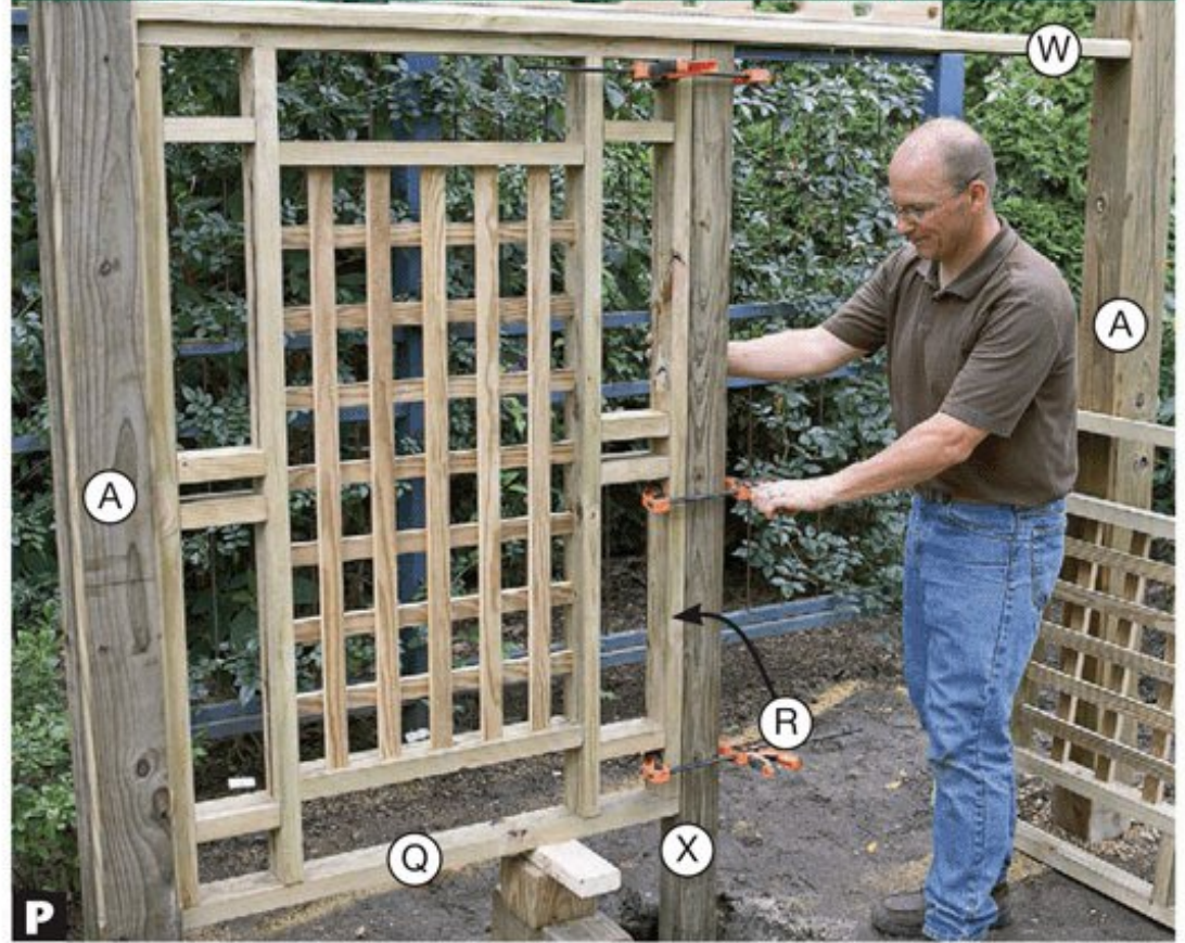
P Clamp the screen post (X) to the upright (R). Screw the upright to the post, then screw the remaining screen (Q-V) in place.
