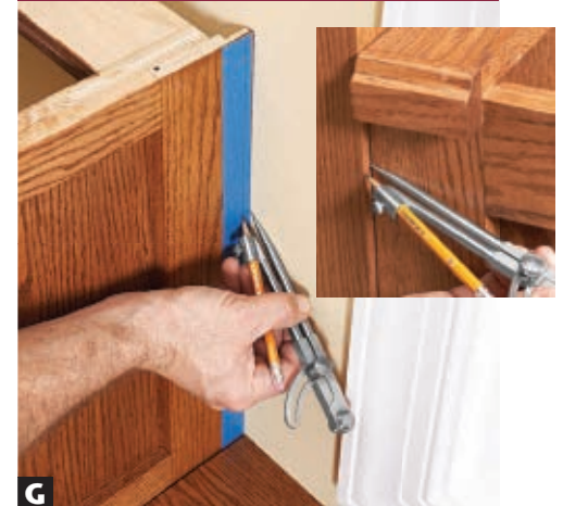
G The difference between the lower cabinet and window-seat depth (inset) equals what you'll remove from the lower-cabinet stile.
