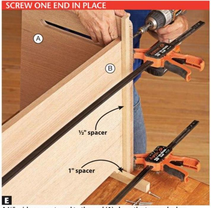
A ½"-wide spacer taped to the end (A) along the tapered edge provides a registration surface for mounting the front and back (B).
