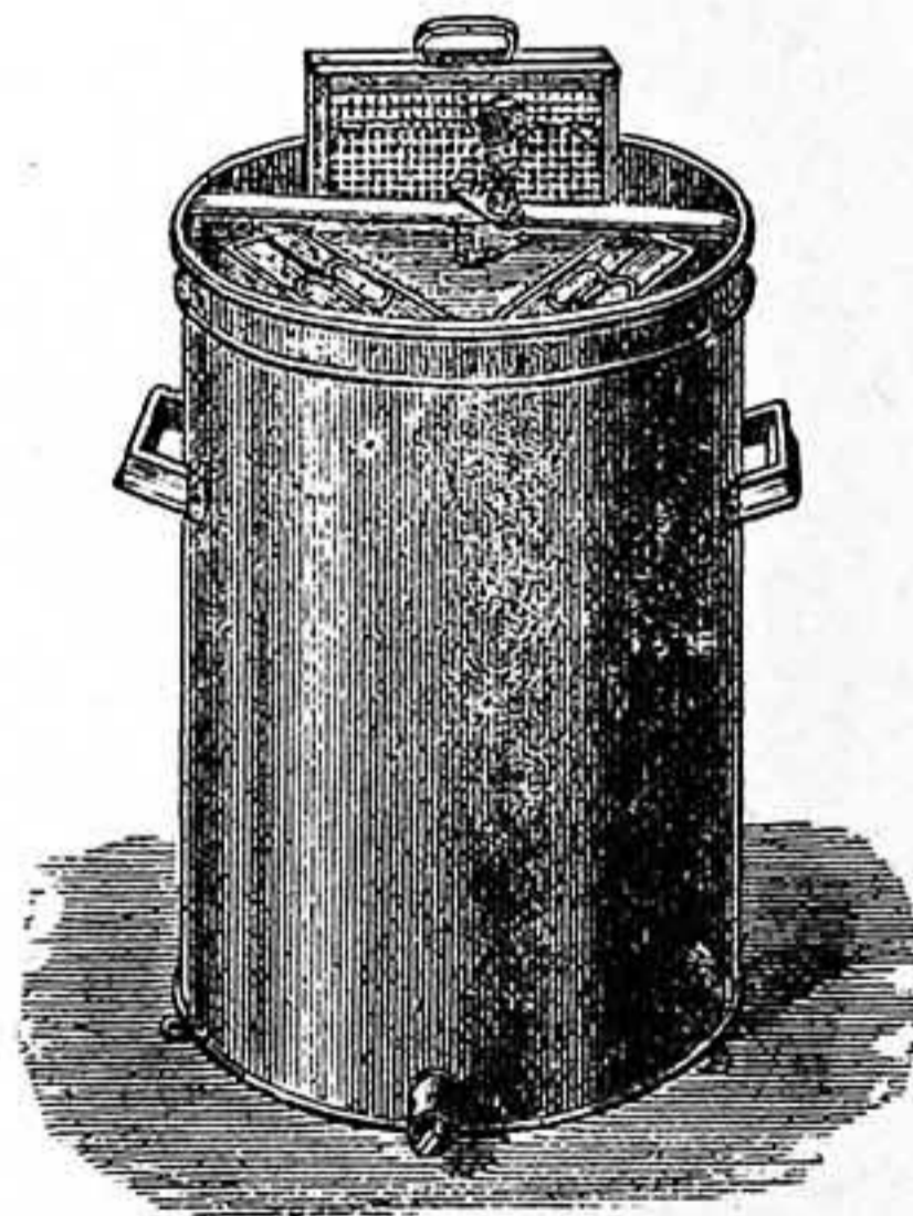
Fig. 2.—Lowth's Bar-Frame Honey Extractor.
